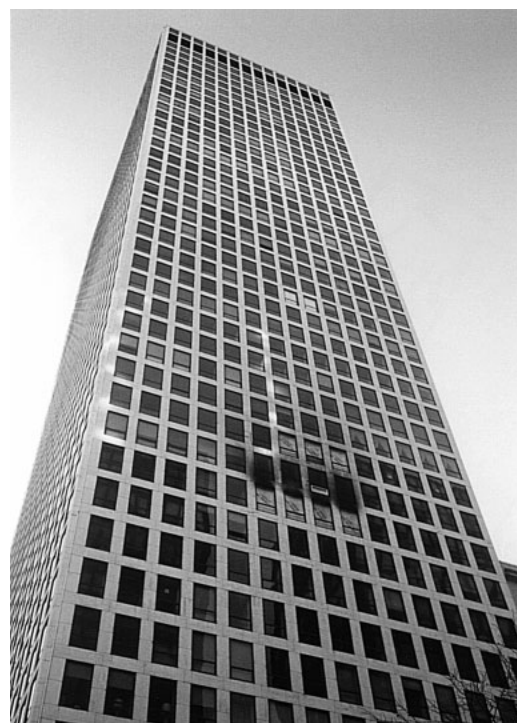
A fire at 260 E. Chestnut Street, on Chicago's Gold Coast in January 2002, resulted in one death and 11 injuries including eight firefighter injuries. The damage was in the millions and some tenants were displaced for more than nine months.
