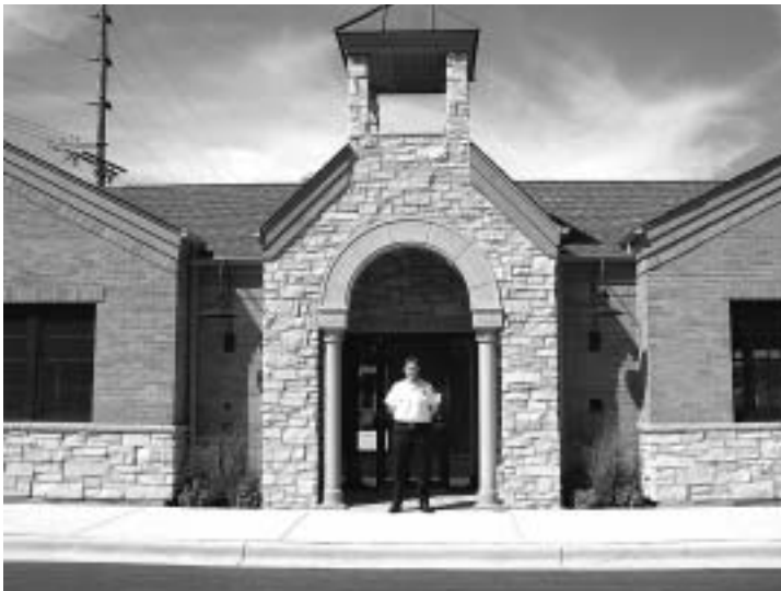
Jeff Lehr stands in front of the new classroom building at the new Lemont Safety Village.
