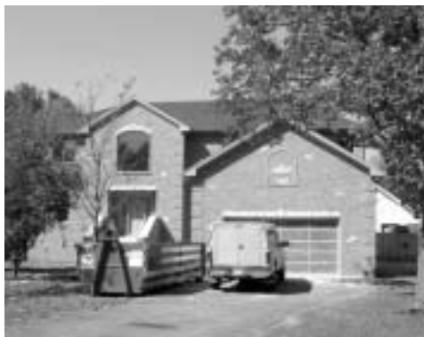
The Redmond home is the first in Prospect Heights with a residential fire sprinkler system. Don Gould, Jr., Fire Chief, Prospect Heights Fire Department.
