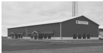
The Frankfort Fire Station and Training Center was retrofit with a fire sprinkler system. The 30,000 sq. ft. building includes a living area, truck bay, training classroom and training prop area.
