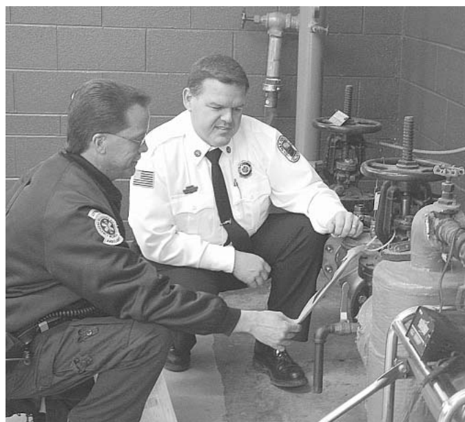
Chief Lindsay Laycoax and firefighter/paramedic Tom Jones, Oak Forest Fire Department, inspect a backflow assembly.
